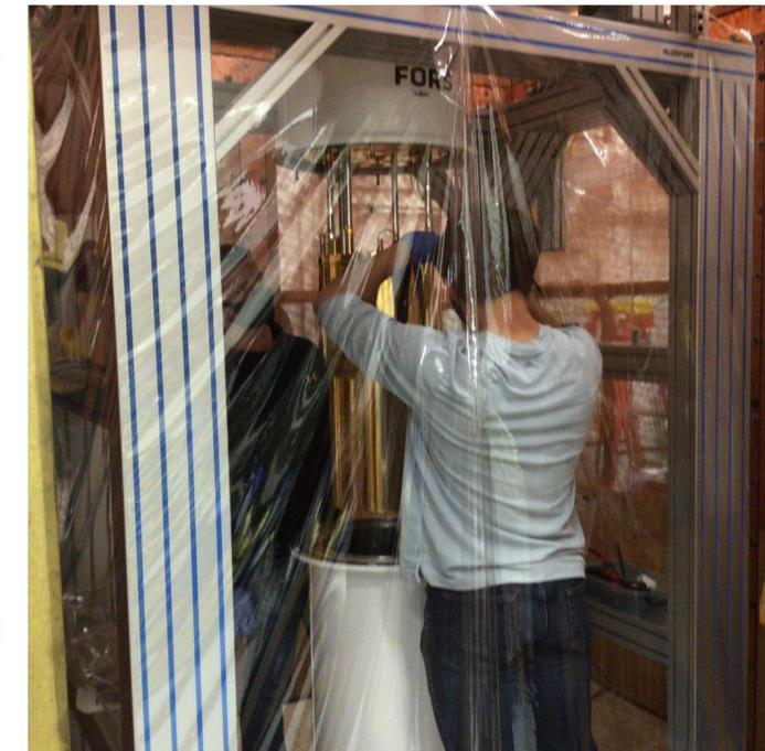
Undergraduates J. Stevic and G. Bimstefer installing optical fibers to pulse cryogenic light detectors
